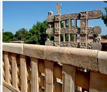
Figure 6: Image showing the fixing detail of stone Baluster and Railing Vedic Railing [10]
