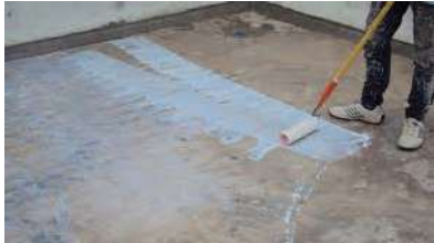
Fig.1. Application of Latex Bonding Agent
